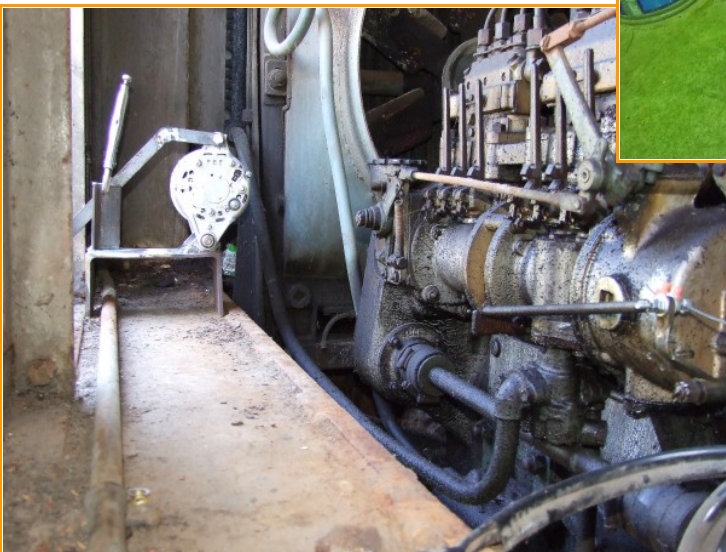
Just about completed. Slotting yet to be done
