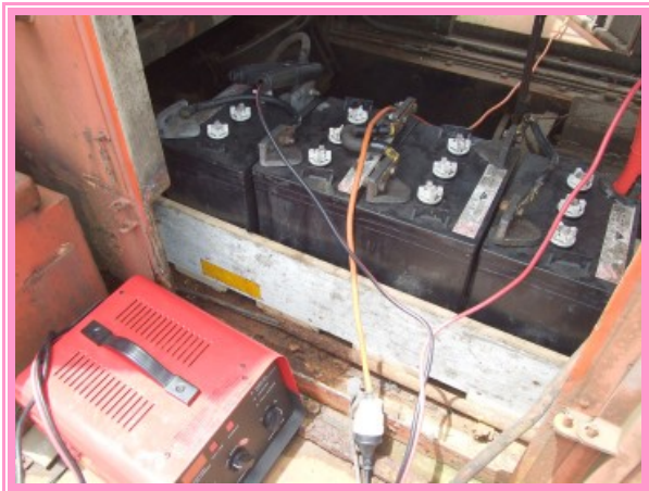
Above;- Lft, Batteries in and connected to each other and on charge Right;- Jim working on the batteries. Photo Denyse B
