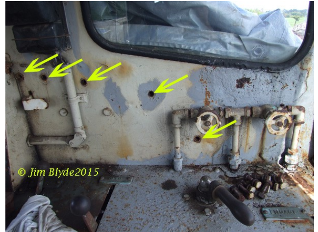
Arrows where the bolts are / were.
