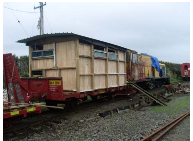
The mobile workshop takes shape
