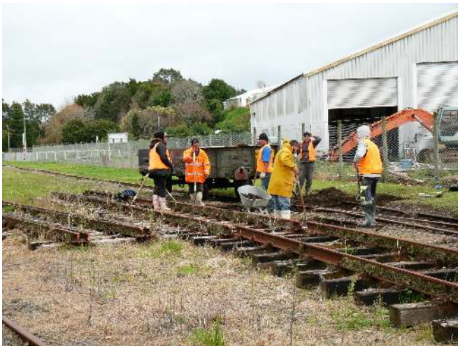
Digging out ballast in Waitara yard
